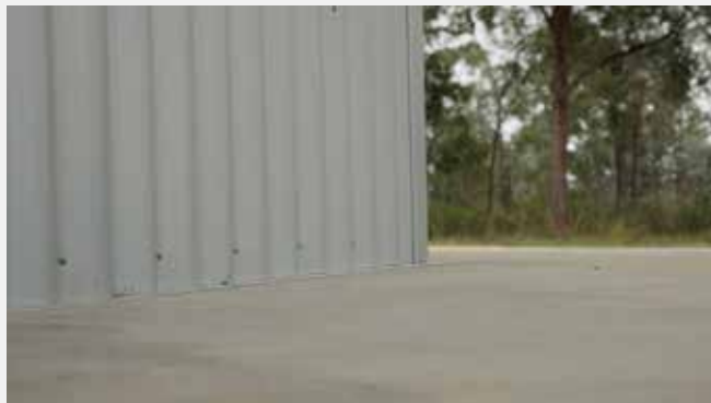
The robust concrete verandah reduces risk of surface fires reaching the home.
